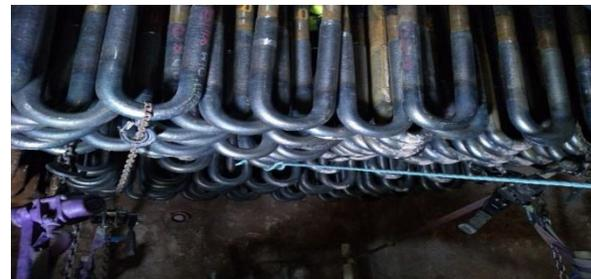
△ Superheater tubes being positioned ready for welding
